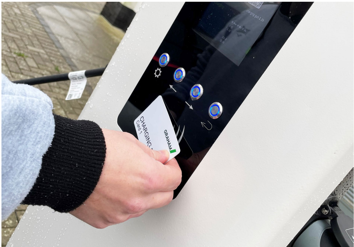
Figure 4 – Electric Vehicle car charging at GRAHAM offices
